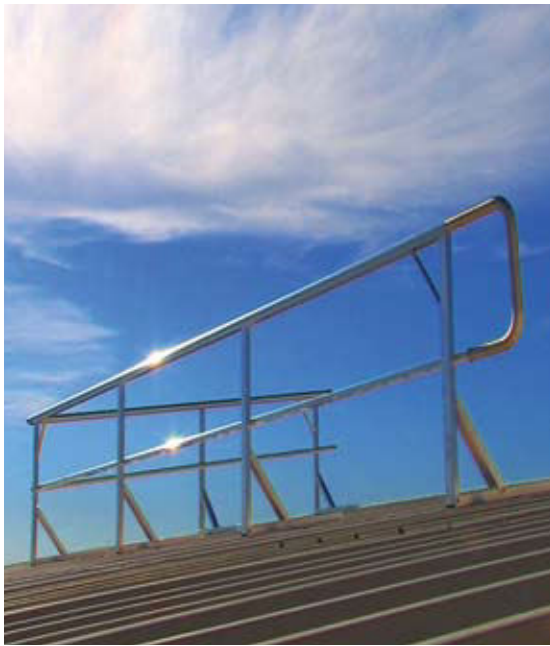
Levelled Walkway with Guardrail one side
